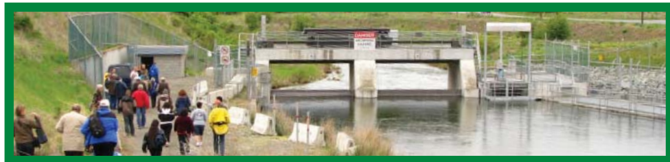
Walking down for a tour of Nicola Dam at the Fraser Assembly.
